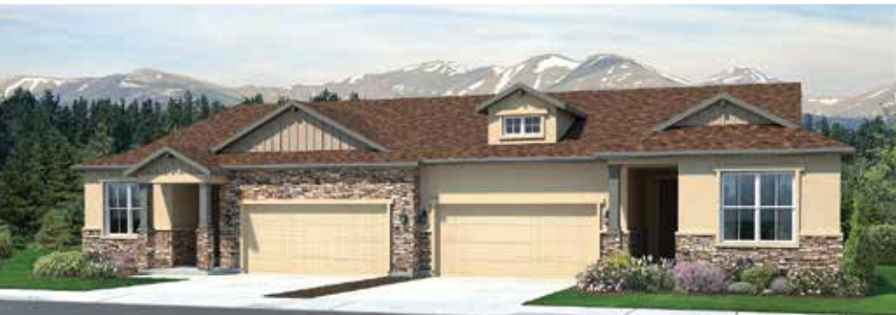
Unit 2B - Building 5121
