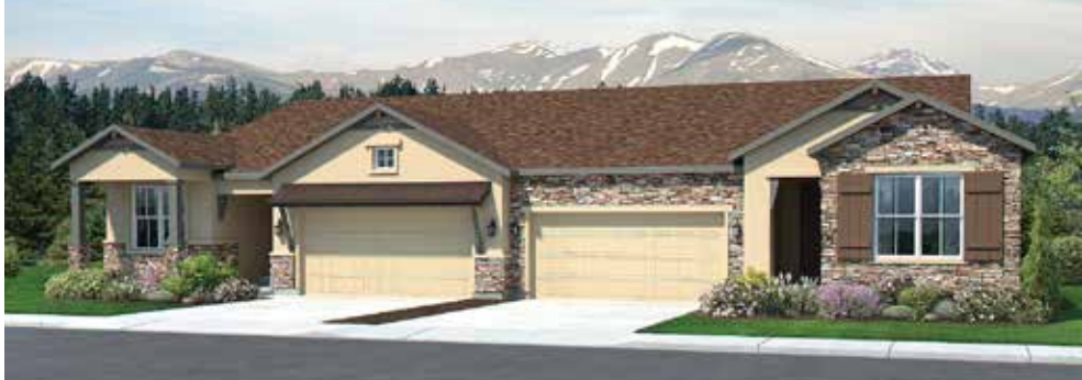
Unit 2A - Building 5121
